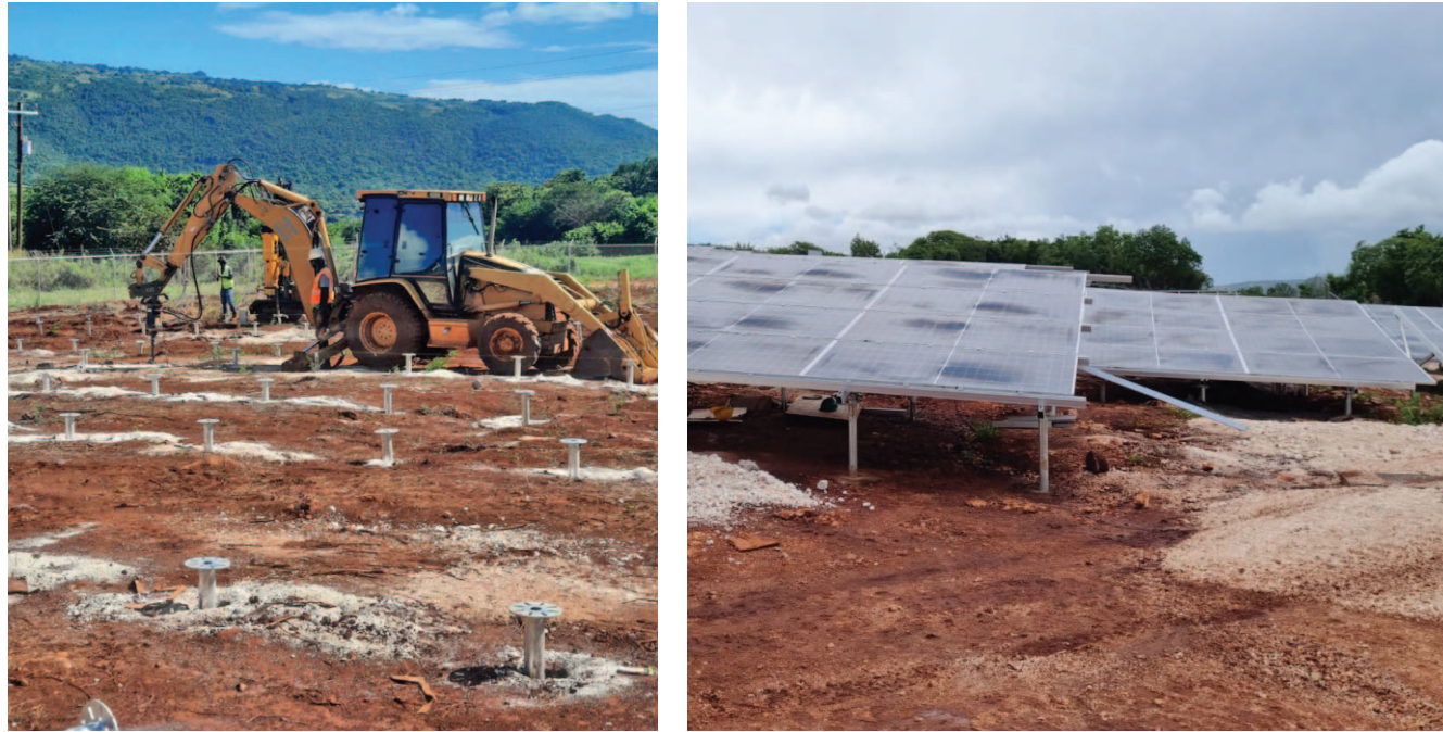
On going solar installation work taking place at Prospect, St. Elizabeth
