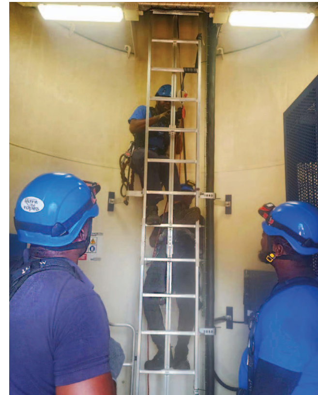
Wigton team members performing repairs on the wind turbines.
